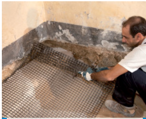
Positioning Mapegrid G 220 alkali-resistant glass fibre reinforcement mesh
