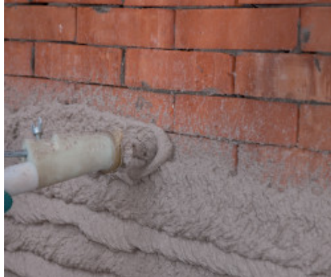
Application of Planitop HDM Restauro by spray on a brick wall
