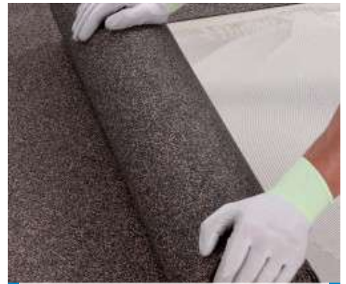
Unroll the sheets of Mapesonic CR on the surfaces to be soundproofed
