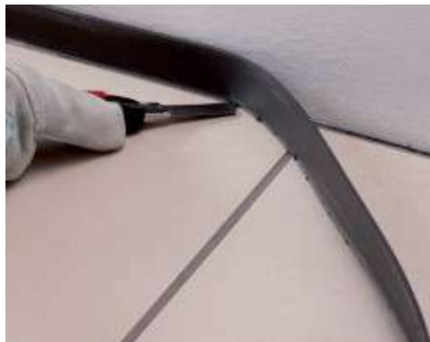
Once the grout has hardened, trim the perimeter of the Mapesonic Strip to remove the excess
