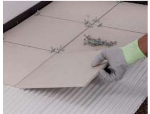
Spread the adhesive on the Mapesonic CR and bond the new floor finish
