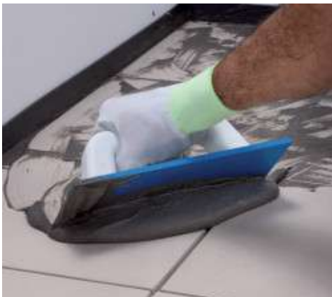
Grout the surface of the room
