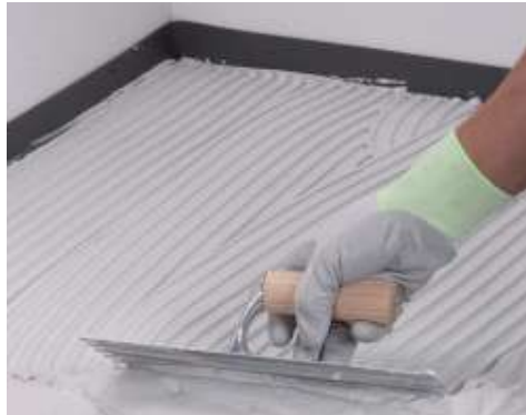
After suitable preparation of the substrate, spread on the adhesive to bond the soundproofing sheets
