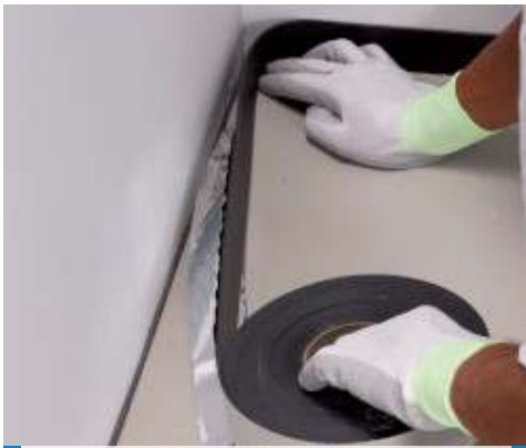
Apply Mapesonic Strip adhesive tape around the perimeter of the room
