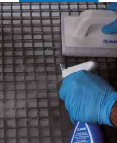
Spraying Kerapoxy Cleaner on the surface requiring cleaning
